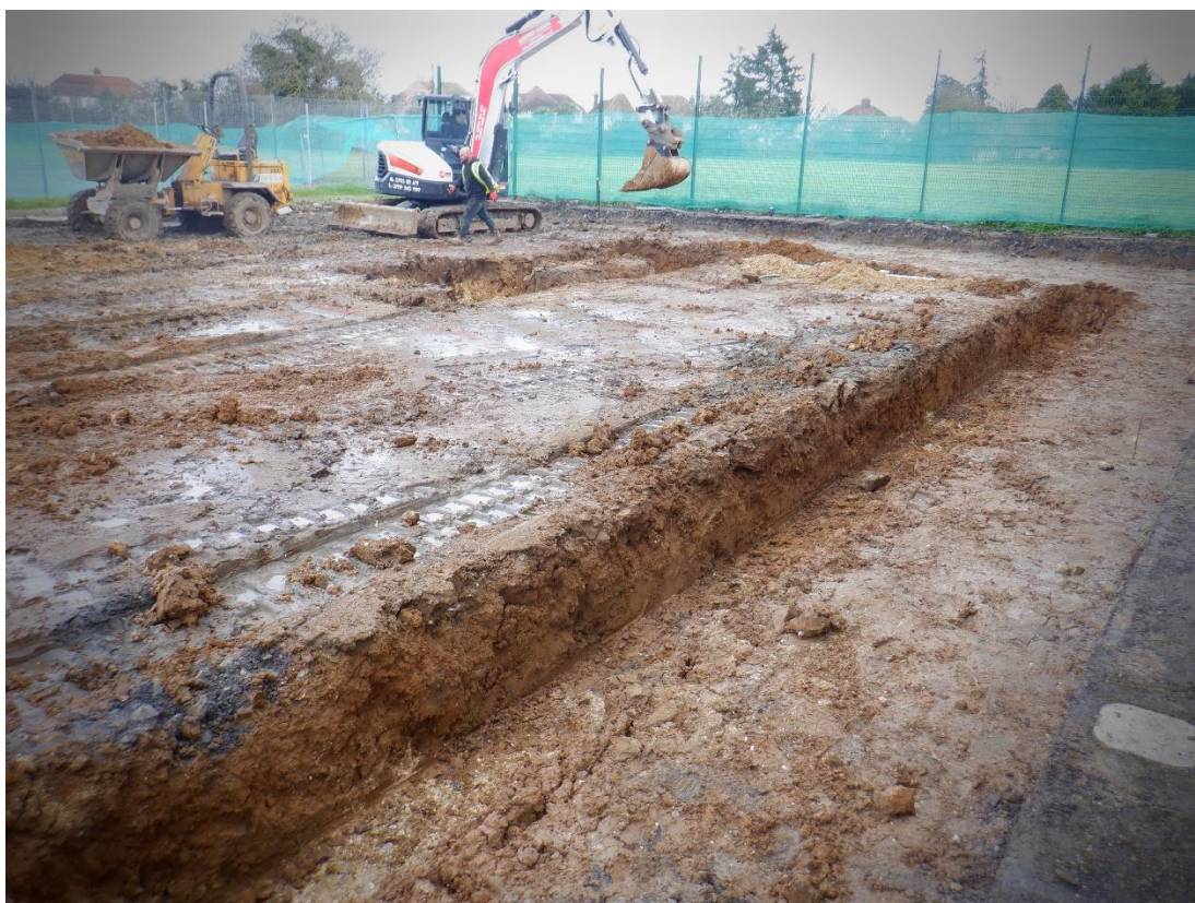
Plate 4. Trenching subsoil (looking SW)
