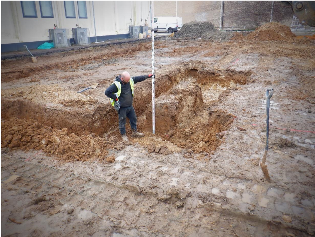
Plate 5. Checking depths of oundation trenches (looking SW)
