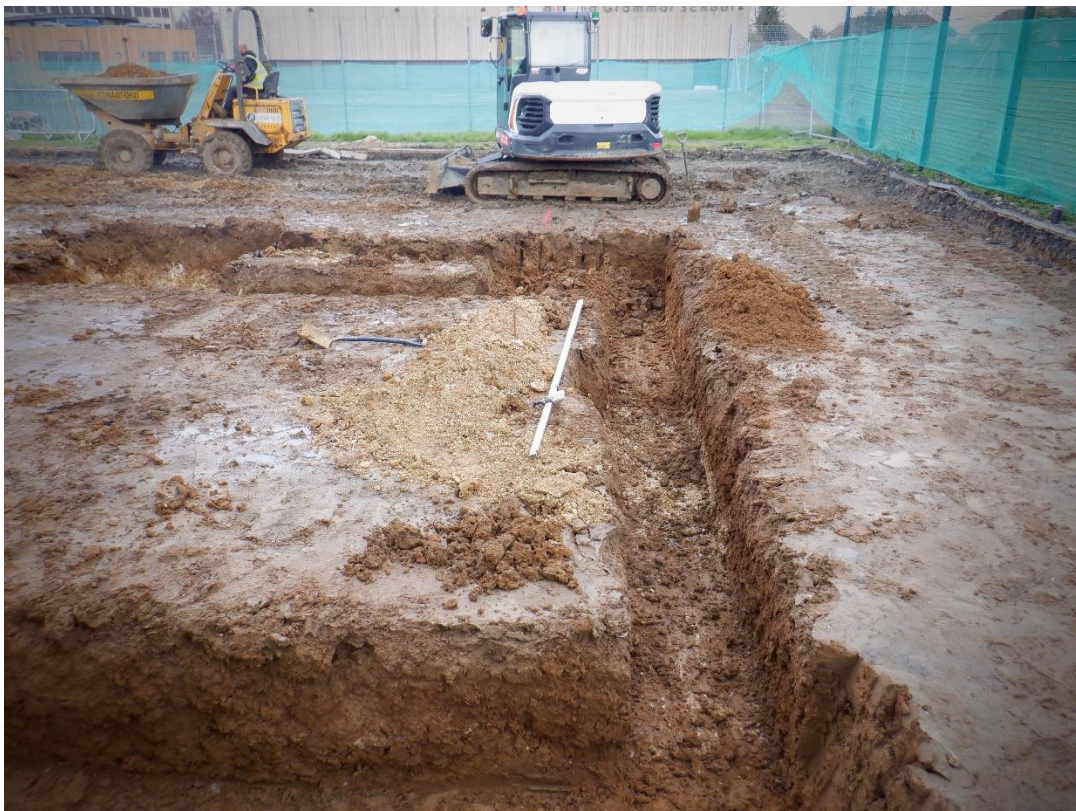
Plate 6. Foundation trenches (looking East)
