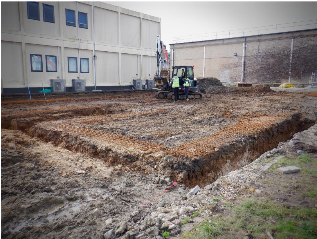
Plate 8. Foundation trenches (Looking SE)
