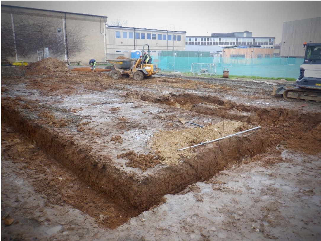
Plate 7. Foundation trenches (Looking SW)
