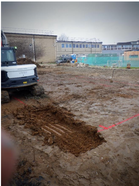
Plate 2. Trenching subsoil (looking SW)
