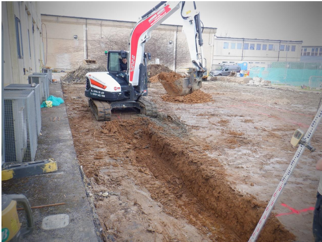
Plate 3. Trenching subsoil (looking South)
