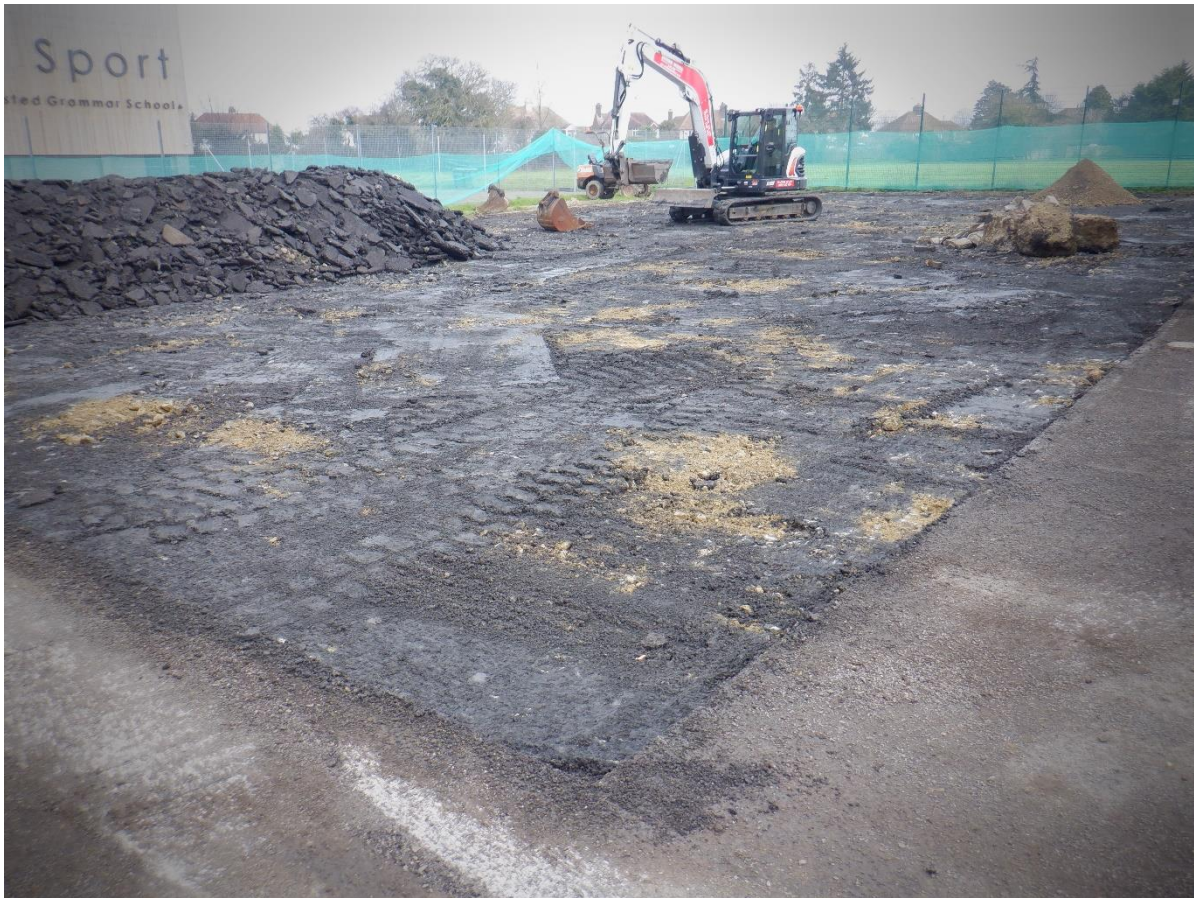
Plate 1. Removing tarmac surfaces (looking NNW)
